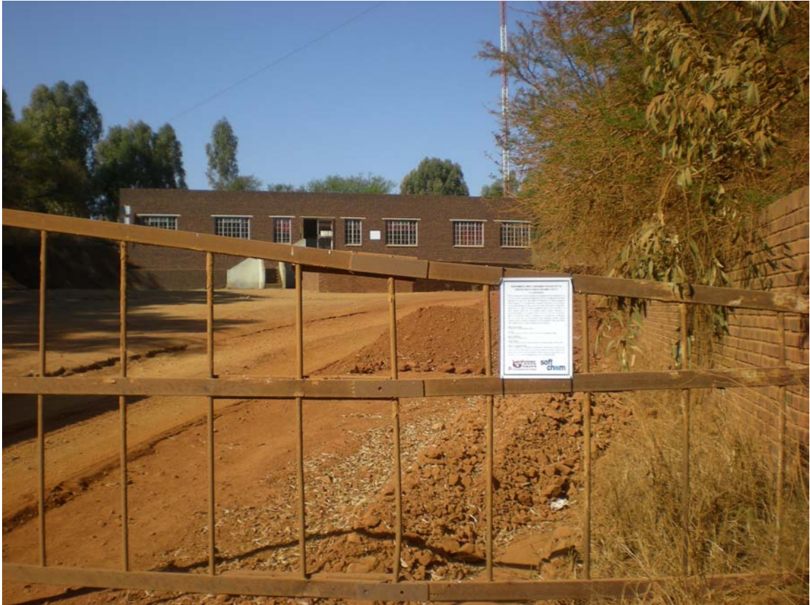
Figure 3 Site notice placed at entrance to site.
